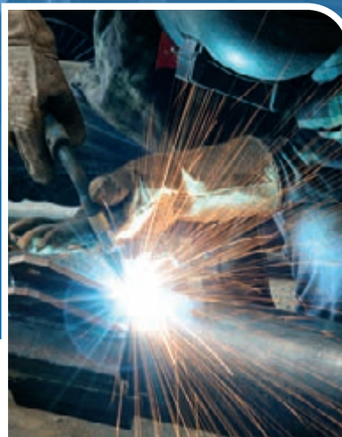
Daviesway's in-house steel fabrication division brings renowned craftsmanship, and makes everything possible.
